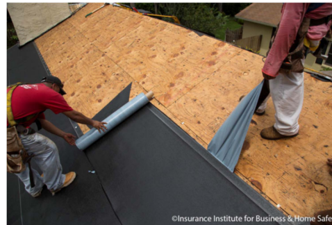
Sample Photo 4: Underlayment “peel-and-stick”
