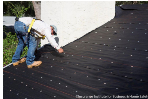
Sample Photo 3: Underlayment Nailing
