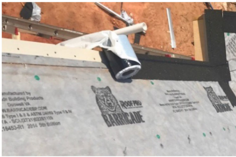
Sample Photo 6: Drip Edge with Self-Adhering Starter Strip
